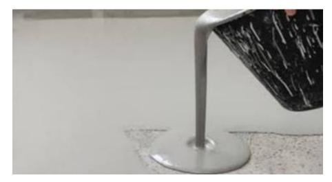
Self-leveling Concrete is a Polymer Modified Cement used to create high compressive smooth Flat surface & the main advantage of Self levelling is, it is faster & Easier than Pouring new Concrete. Selfleveling thickness is usually considered from 3mm to 10mm as per client Work Requirement
