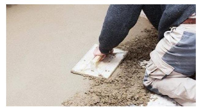
Bonded Screed – This type of screed where the Screed layer is bonded fully to the substrate using a primer or bonding agent. This type of screed is ideal for thinner section screeds where heavy loading is expected. A bonded screed is generally of15– 30mm thick.
