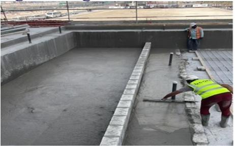
**Cellular concrete or Light Weight Foam concrete** is a type of porous concrete, Basically Foam concrete is a mixture of cement, water and foaming agent. When the foaming agent is diluted with water and air, further it is mixed into the cement slurry.
